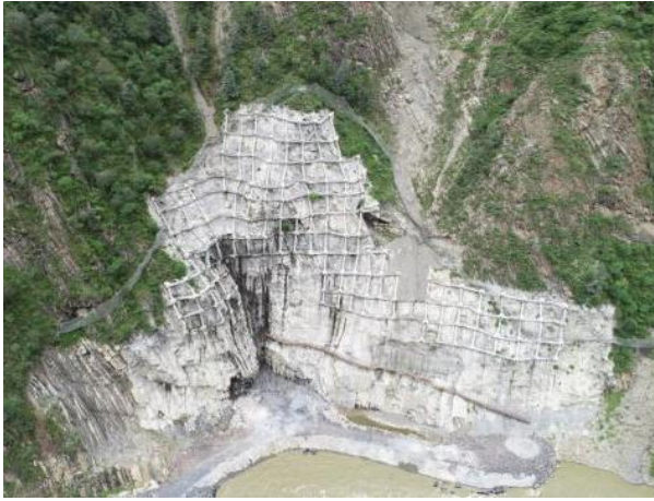
导流洞进口边坡支护 (2018.9)
