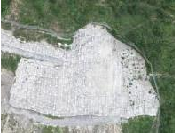
导流洞出口边坡支护 (2019.9)
